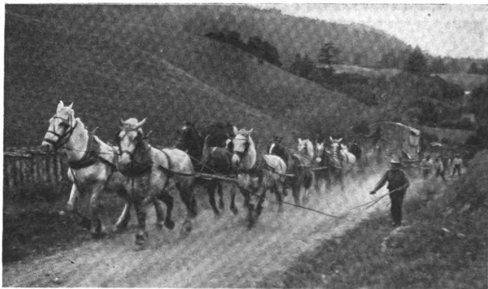
The powerful motor generators on the road to Bolinas. This picture shows the character of the country and the grades over which the heavy machinery had to be transported
