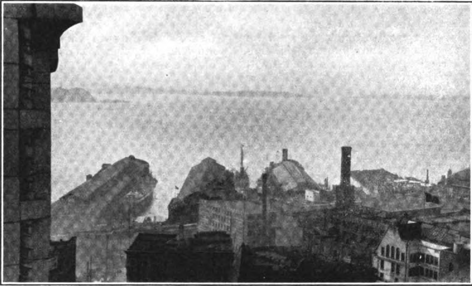
The Seattle waterfront, viewed from the Marconi offices in a new skyscraper.
