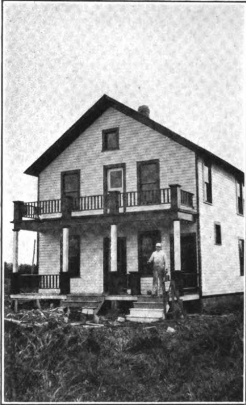
Living quarters at Ketchikan and Juneau have been designed with special provisions for the comfort of the Alaskan operators
